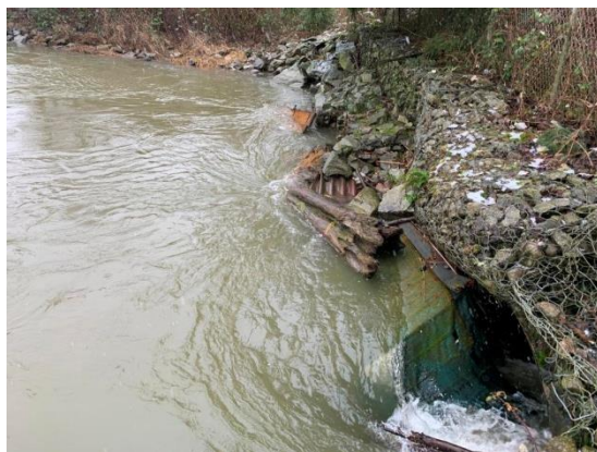
Culverts after CPR left
